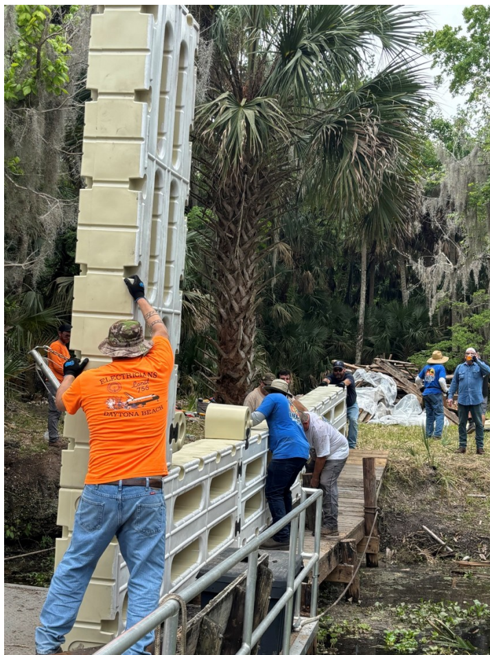
Above: Crew replaced the old Tick Island dock with a new floating dock.
