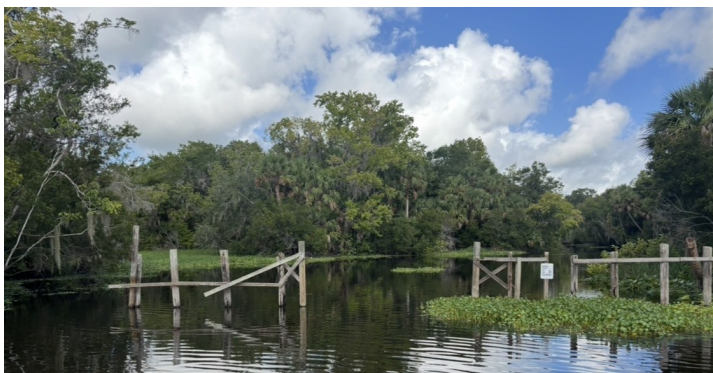
Below/Right: Crews replaced the boards and restabilized the fence at the entrance to Tick Island.
